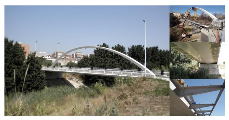
The arch bridge over Picassent Gorge consists of a single steel arch of 51,50 m span with a composite deck connected to the arch by means of steel hangers.
